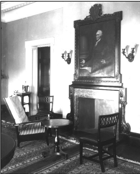
Room 3330 shortly after 1910 remodeling
