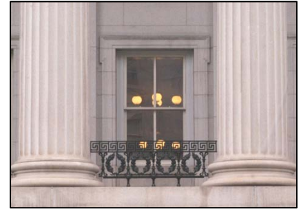
Reproduction of 1842 Original Railing Photo courtesy of Don Adams
